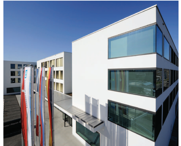
Endress+Hauser's head offices in Reinach, Switzerland
